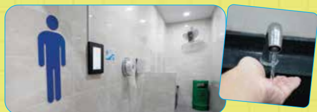
New washrooms come equipped with auto-flush features for urinals and toilet bowls and motion-sensored water taps.
