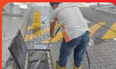
Flushing of Drains
