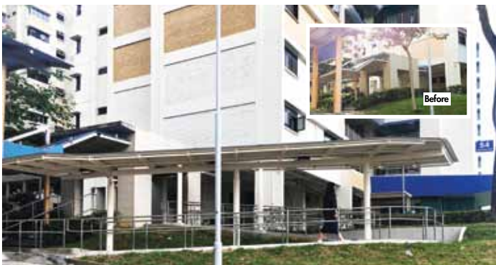
Construction of Barrier-Free Access ramp (BFA) at Blk 50 Telok Blangah Drive near lift A to LTA linkway
