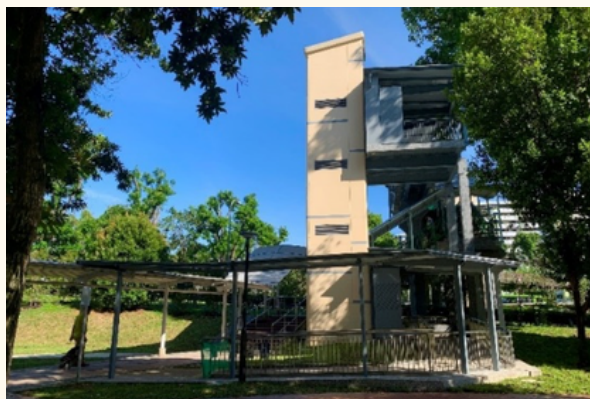
Completed lift shaft near Blk 506 West Coast Drive, across AYE leading to Clementi Town Centre
