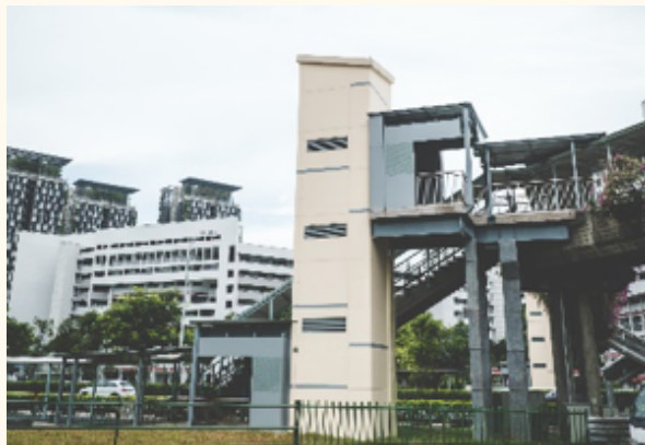
Completed lift shaft near Blk 610 Clementi West St 1
