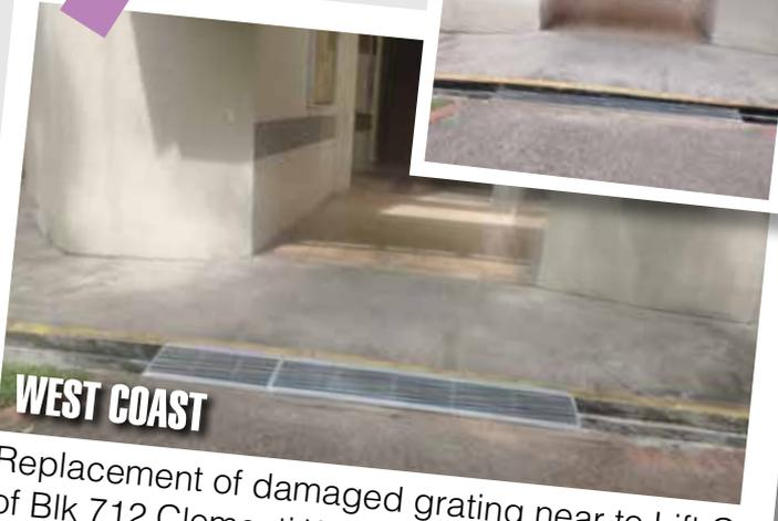
Replacement of damaged grating near to Lift C of Blk 712 Clementi West St 2
