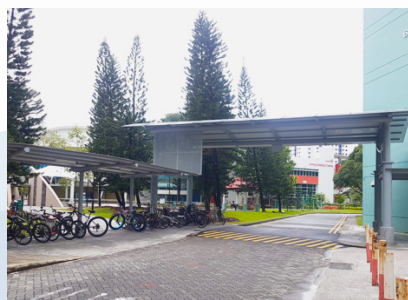
New Covered Linkway near Blk 688 Jurong West Central 1
