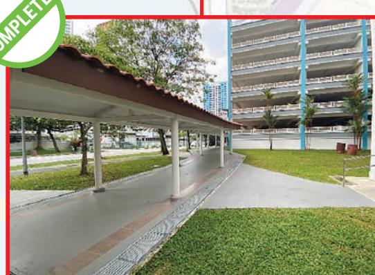
New Covered Linkway From Blk 30 - 63A Teban Gardens Road
