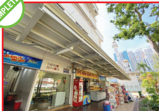
New Covered Walkway at Shopfront for Blk 49 & 54 Teban Gardens Road
