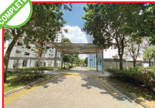
New High & Low Covered Linkway from Blk 32 - 64 Teban Gardens Road
