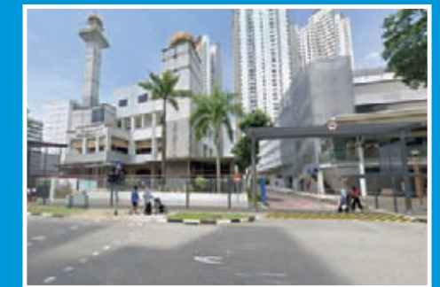
Construction Of High / Low Covered Linkway Location: Blk 49 - 61 Teban Gardens Road Estimated Completion: 3rd Quarter 2023
