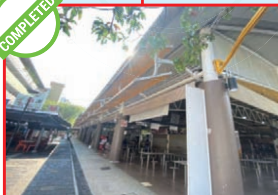
Completed Repairs and Redecoration Works at Blk 37A Market & Food Centre
