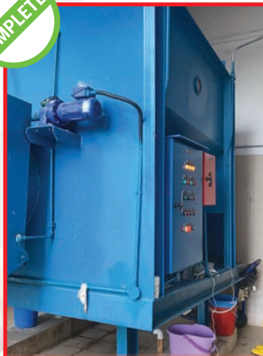
Replacement of Refuse Handling Equipment for Blks 60, 62 - 65 Teban Gardens
