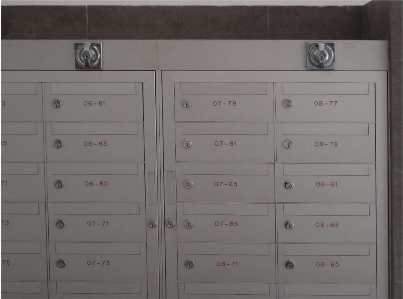
ALL LETTERBOXES TO BE UPGRADED TO CURRENT STANDARD INCLUDING INCREASED FONT SIZE AND IMPROVED LIGHTING
