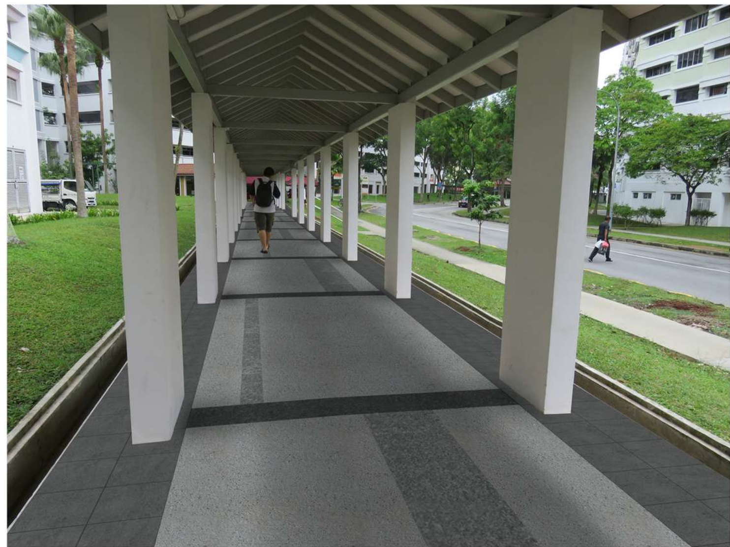
MODIFICATION OF EXISTING LINKWAY ALONG JURONG WEST ST 81 IN RESPONSE TO RESIDENTS' FEEDBACK OF SLIPPERY FLOOR DURING RAIN CHANGE OF EXISTING FLOOR TILES TO MORE SLIP RESISTANT FINISHES
