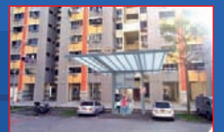
Construction of Drop-off Porch with Low Covered Linkway Estimated Completion: June 2023 Location: Blk 730
