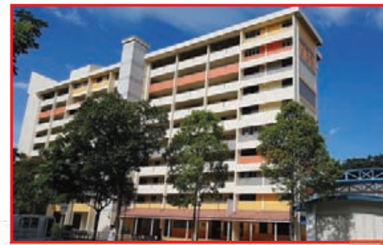
Completed Repairs and Redecoration Work at Blk 731
