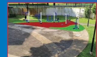
Construction of Elderly Fitness Corner Estimated Completion: June 2023 Location: Near Blk 612
