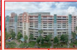
Completed Repairs and Redecoration Work at Blk 706
