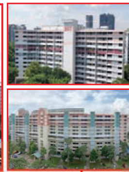
Completed Repairs and Redecoration Work at Blk 605
