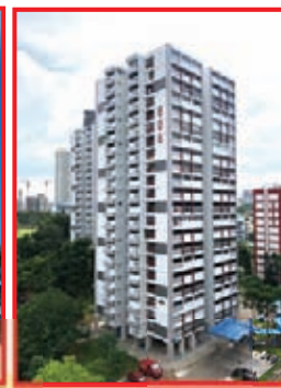
Completed Repairs and Redecoration Work at Blk 606
