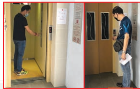
Completed Lift Enhancement at Blk 603
