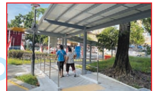
New Sheltered Barrier Free Access Ramp at Blk 601
