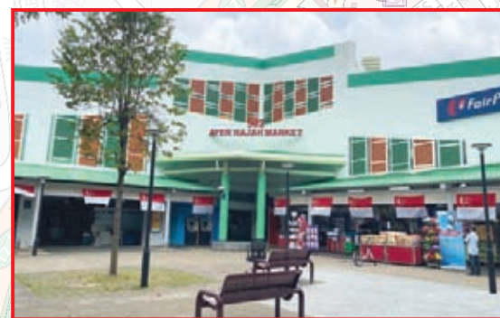
Repairs and Redecoration Work for Ayer Rajah Market
