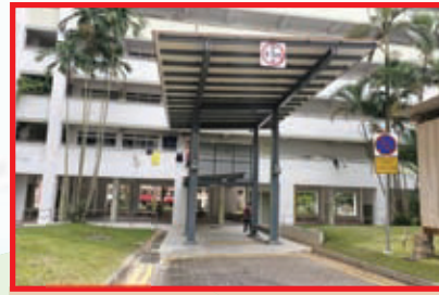
New Drop-off Porch at Blk 832
