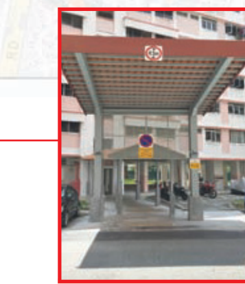
New Drop-off Porch at Blk 979
