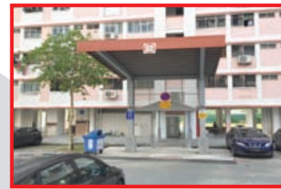
New Drop-off Porch at Blk 980
