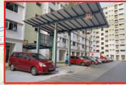
New Drop-off Porch at Blk 812
