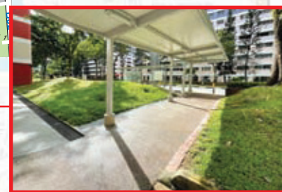
New Covered Linkway from Blk 934 - Bus Stop
