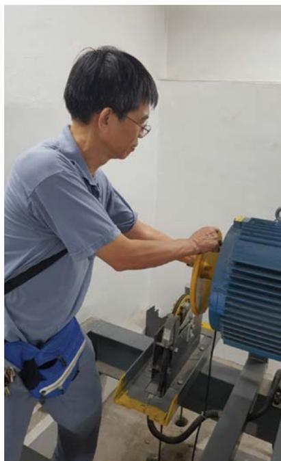
For lifts with motor room, LRO will manually wind the lift car to the next nearest landing.
