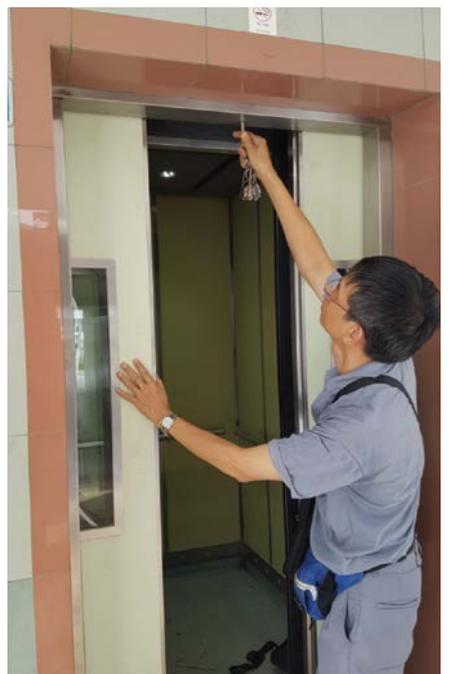
LRO opening the lift doors to release the trapped passengers.
