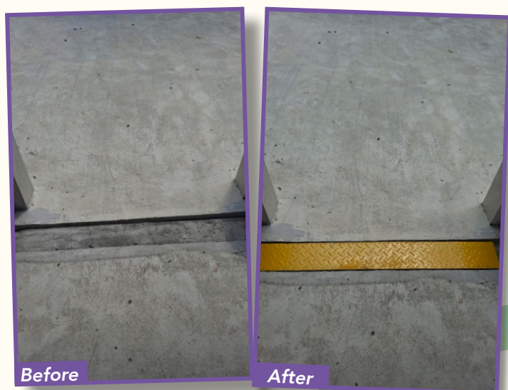
Installation of Anti-slip Plates at Block 25 Teban Gardens
