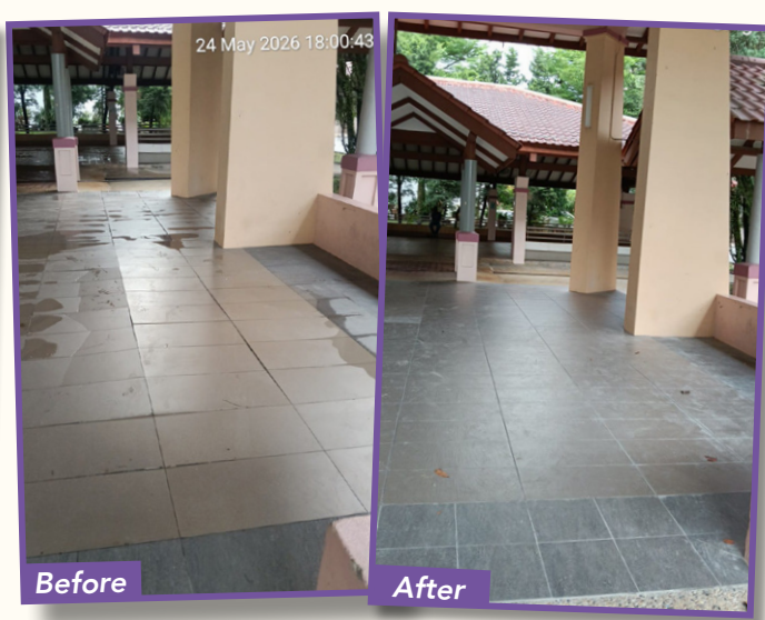
Replacement of Damaged Tiles at Block 120 Ho Ching Road
